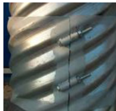
Geometric properties of coupling bands are adjusted to the geometry of HelCor® pipes.
